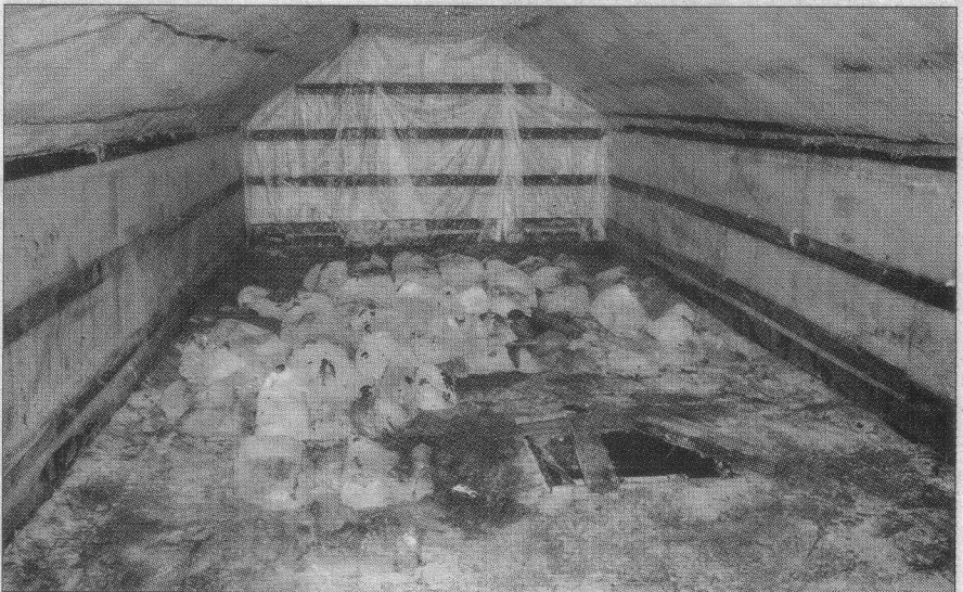
At Smyrna Mills, cheese is kept cold without electricity. An insulated room above the cheese is filled each January with ice cut from a near by pond. Trap doors circulate the cold air as needed.
